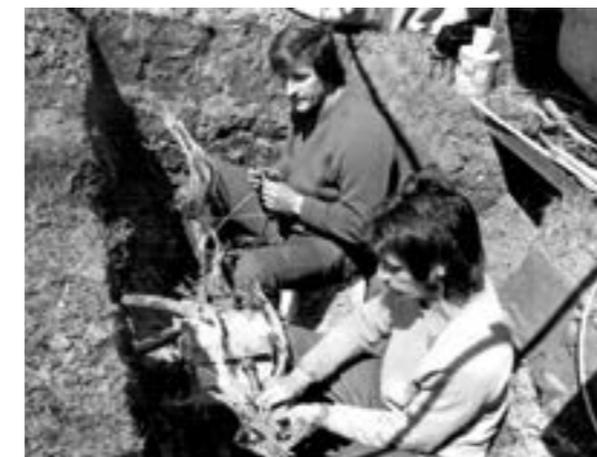
Muffenmontage am Telefonerdkabel 1973
